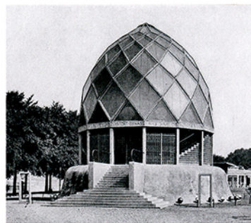
Glass Pavilion, designed by Bruno Taut for the Deutscher Werkbund Exhibition, Cologne, Germany, 1914
